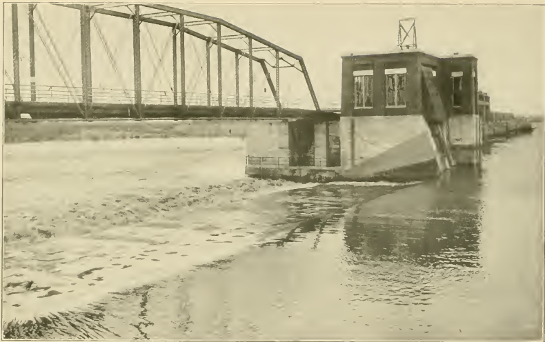
A VIEW OF THE CONTROLLING WORKS ON THE DRAINAGE CANAL Bear trap dam at Lockport looking down stream.
