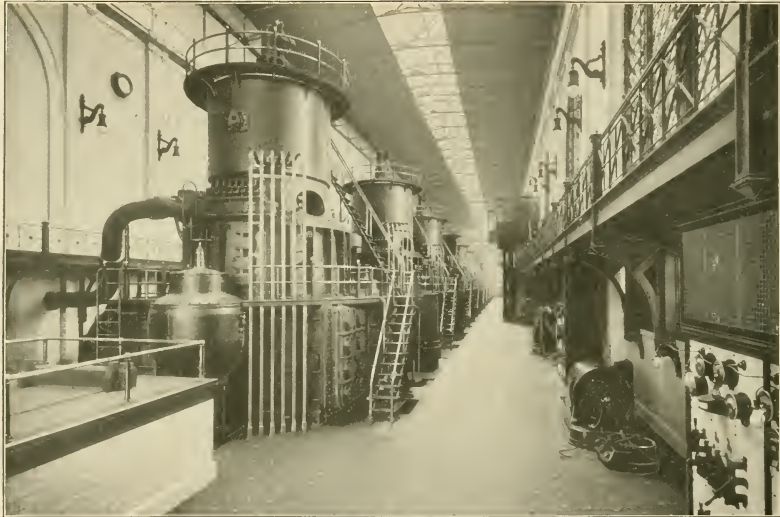
COMMONWEALTH EDISON COMPANY Electric plant showing ten Turbo-Generators in Fisk Street Station.
